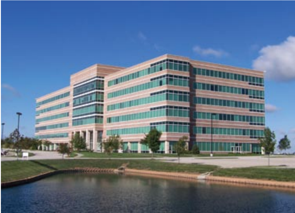
The Ambassador building is Class A office space the airport acquired in September 2006.
