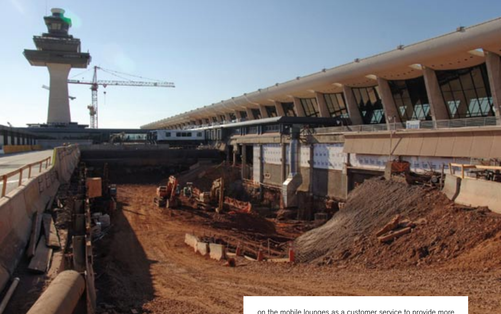
Major excavation efforts enabled ample space for AeroTrain stations.
